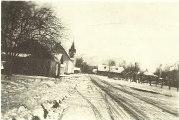
Above: The church building, pre-1929, facing east and sitting across the street from its present location (courtesy of Mrs. Faith Callahan).
