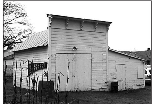
2006 photo of building, on the alley side of the Bronemann property. The lean-to on the right is a later addition and need not be saved.
